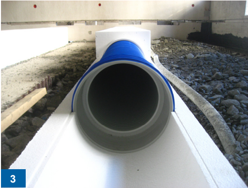
Measure where to place the sleeve and cut the inset
